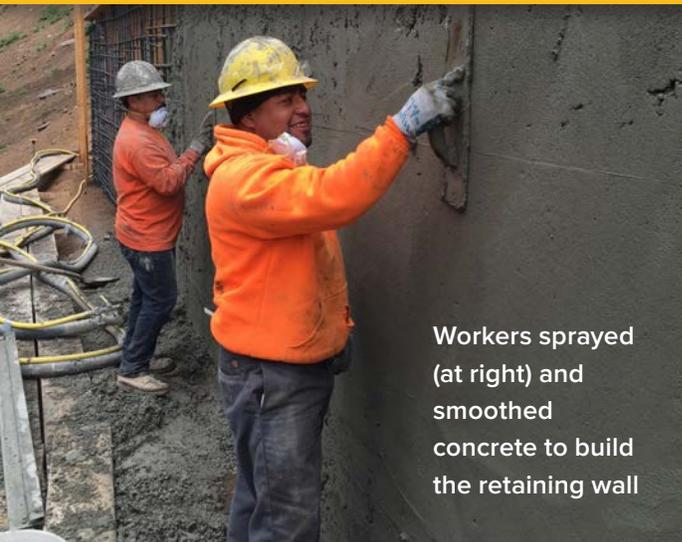
Workers sprayed (at right) and smoothed concrete to build the retaining wall
